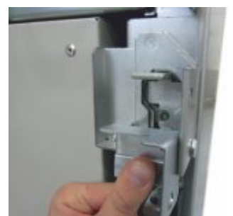
Socket for operation with earthing switch
