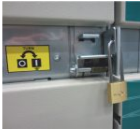
The earthing switch can be locked with a padlock
