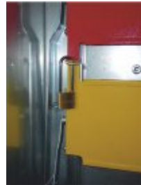
Live shutters can be securely locked in the open and closed positions with a padlock
