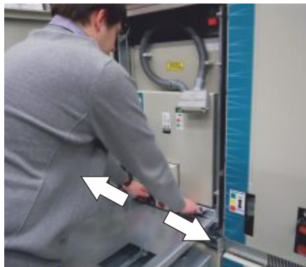
Push DOU into the compartment until it sets into place
