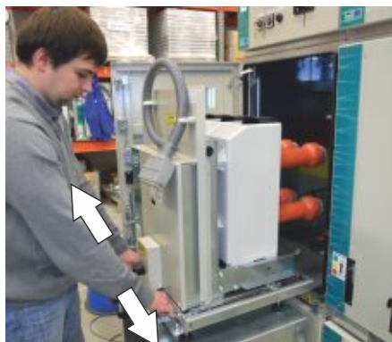
Pull DOU backward on the trolley ramp until the DOU fixing blades click
