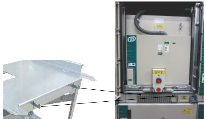
Position of trolley guides directed into the guide openings
