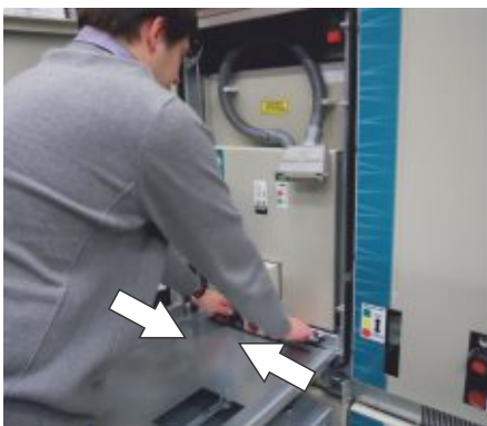
Slide 2 handles simultaneously to the middle
