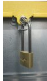
Live shutters can be securely locked in the open and closed positions with a padlock
