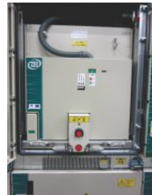
DOU is in the test position
